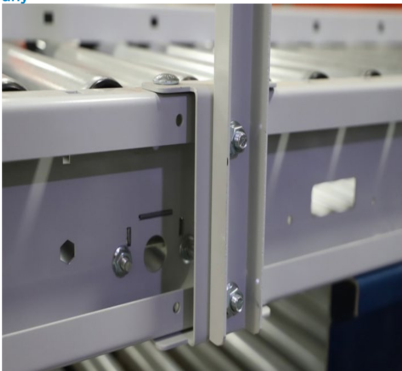
Figure 36: Secured Cable Mast
