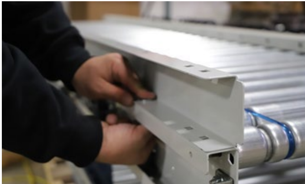
Figure 18: Placement of Guide Rail on Flange
