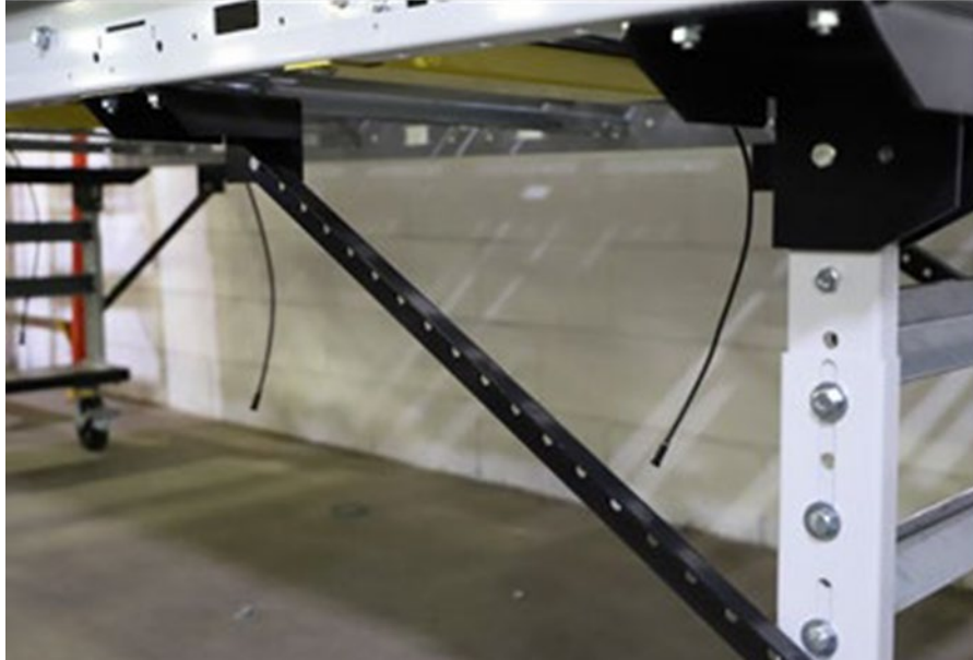
Figure 8: Installing Sway Brace Kit
